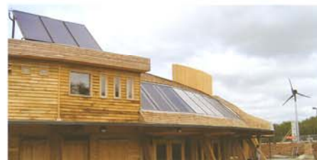
The Centre's solar panels (top left, centre) and wind turbine (right)
